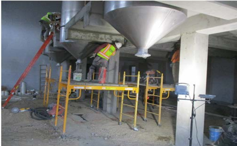
Figure 4 – Installation of solids thickening equipment in the new Solids Handling Facility
