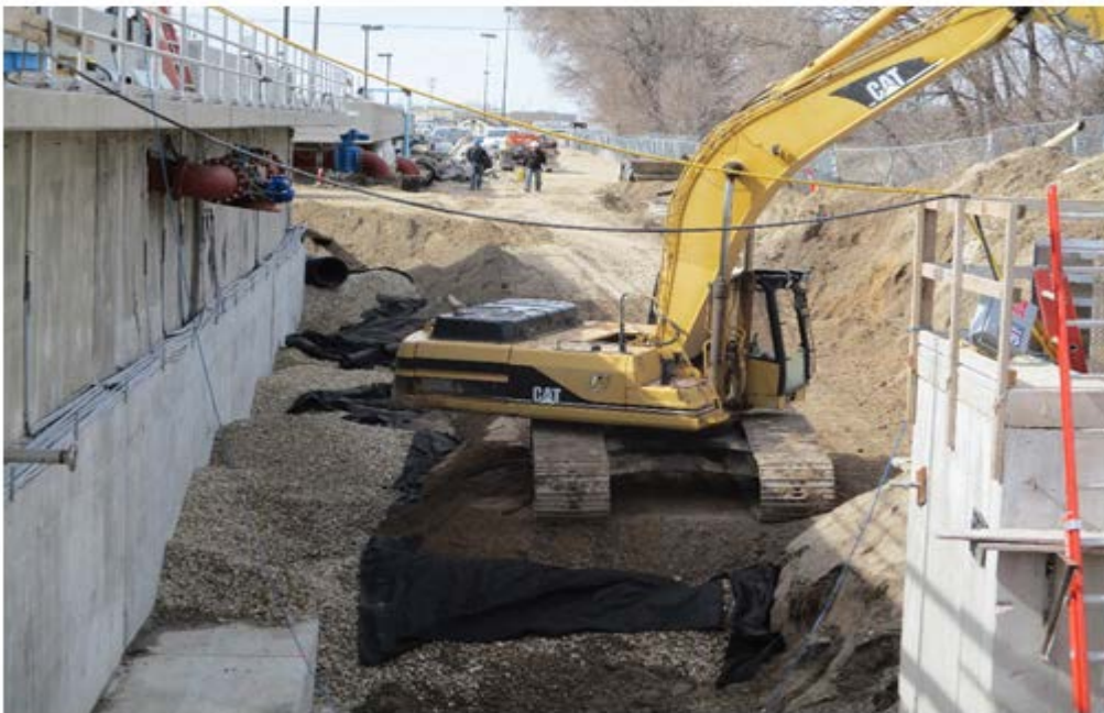
Figure 2 – Backfilling activities on the northern side of the Aeration Basin No. 3
