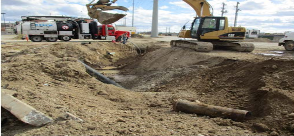
Figure 3 – Excavation for yard piping to the Solids Handling Facility
