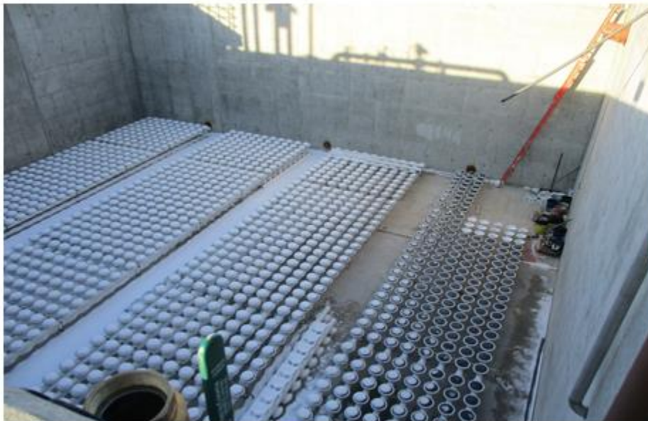
Figure 2 – Diffuser system installation in the new Aeration Basin No. 3.
