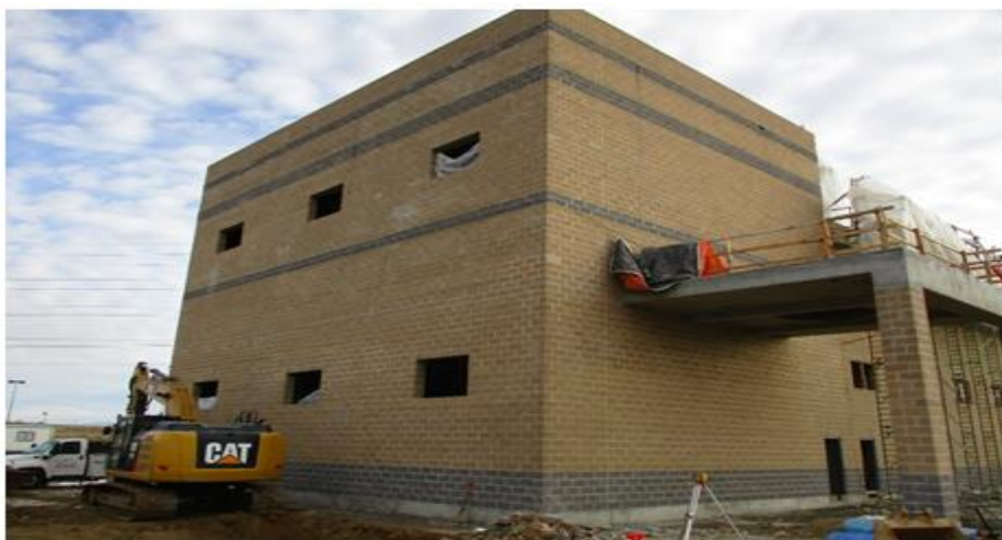
Figure 3 – Masonry progress at the new Solids Handling Facility
