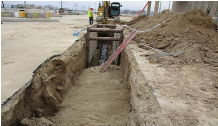
Figure 4 – Underground piping installation to support new Solids Handling Facility
