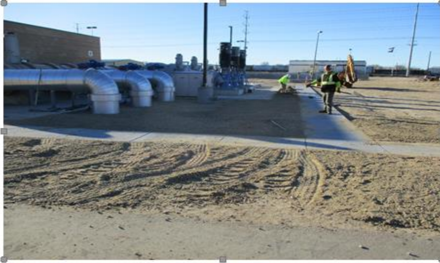
Figure 1 – Site grading around the new Primary Effluent Pump Station
